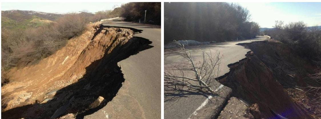
**Figure 1. Landslides on the area of the road Tashkent – Chimgan, (March, 2017 y.)**
